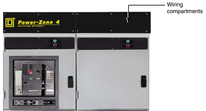
Figure 9: Removing the Wiring Compartment Covers
